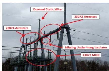
Damaged A-Frame
