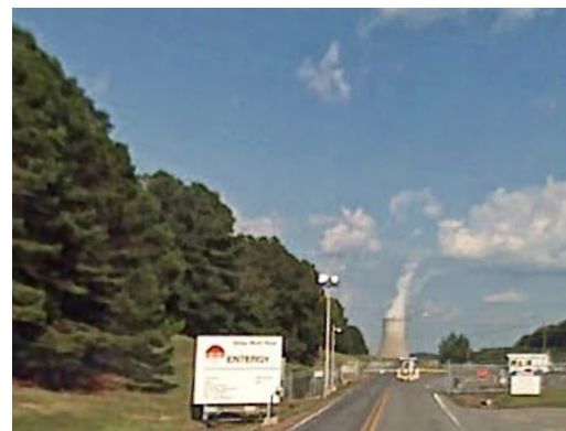
White Bluff Power Plant (Source: Google)
